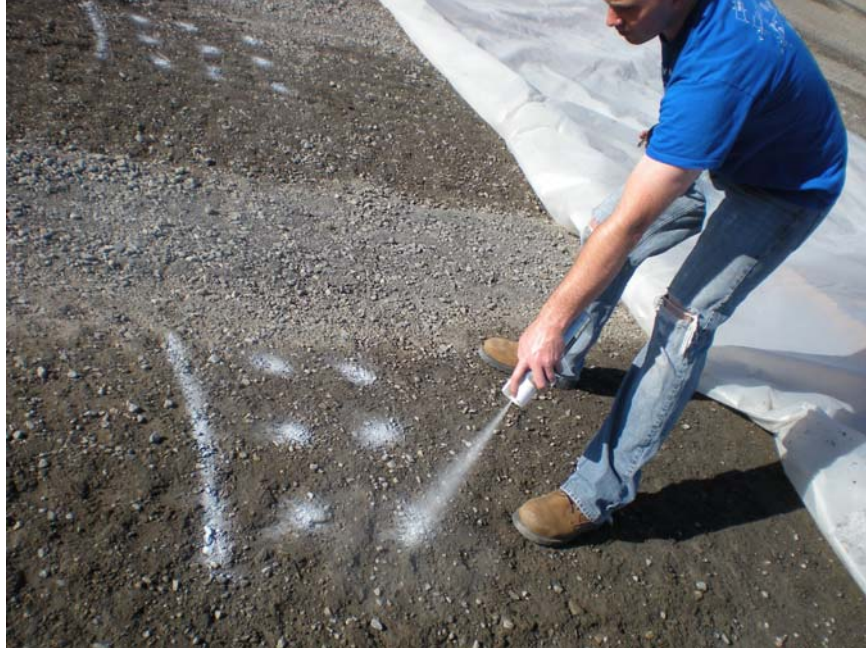
FIGURE 3.2 Marking of operator test locations.
